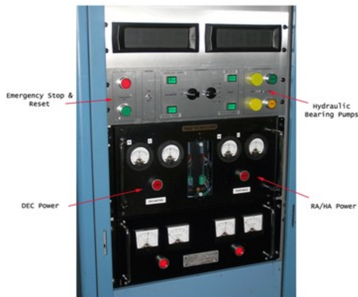
Looking into right side of old control room
